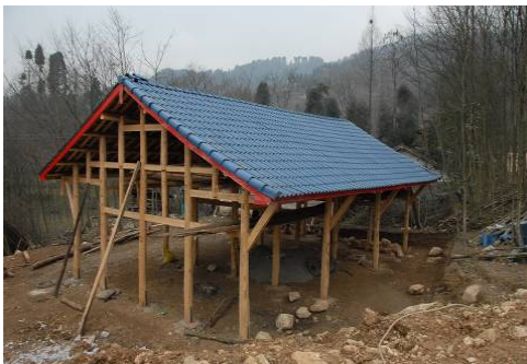
Fig. 2 traditional timber frame structure
